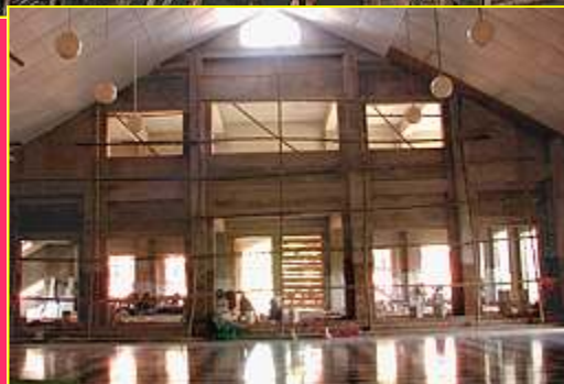
View of the new extension from the platform in front of Pancha-tattva altar.
