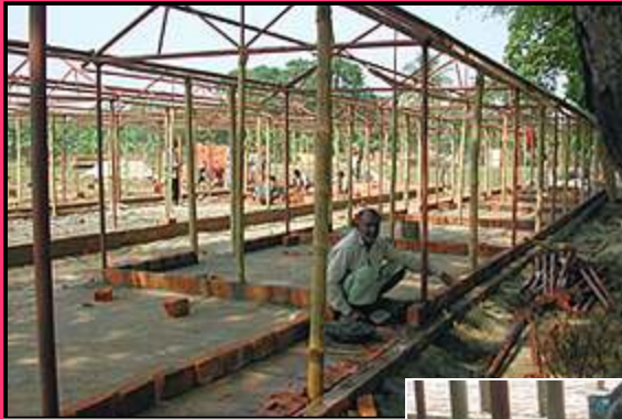
Photos: bamboo rooms under construction.
