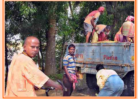
Temple Comander, Kesava Prabhu, supervising the work on the sand bags
